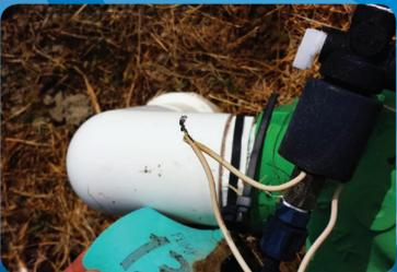
Poor wiring will result in the coil only operating intermittently.
