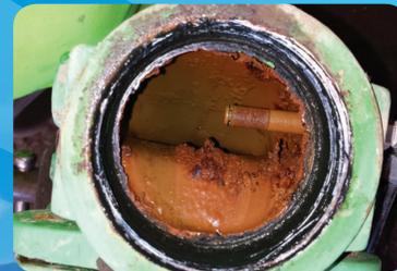
Sediment buildup and corrosion impedes the performance of the valve.
