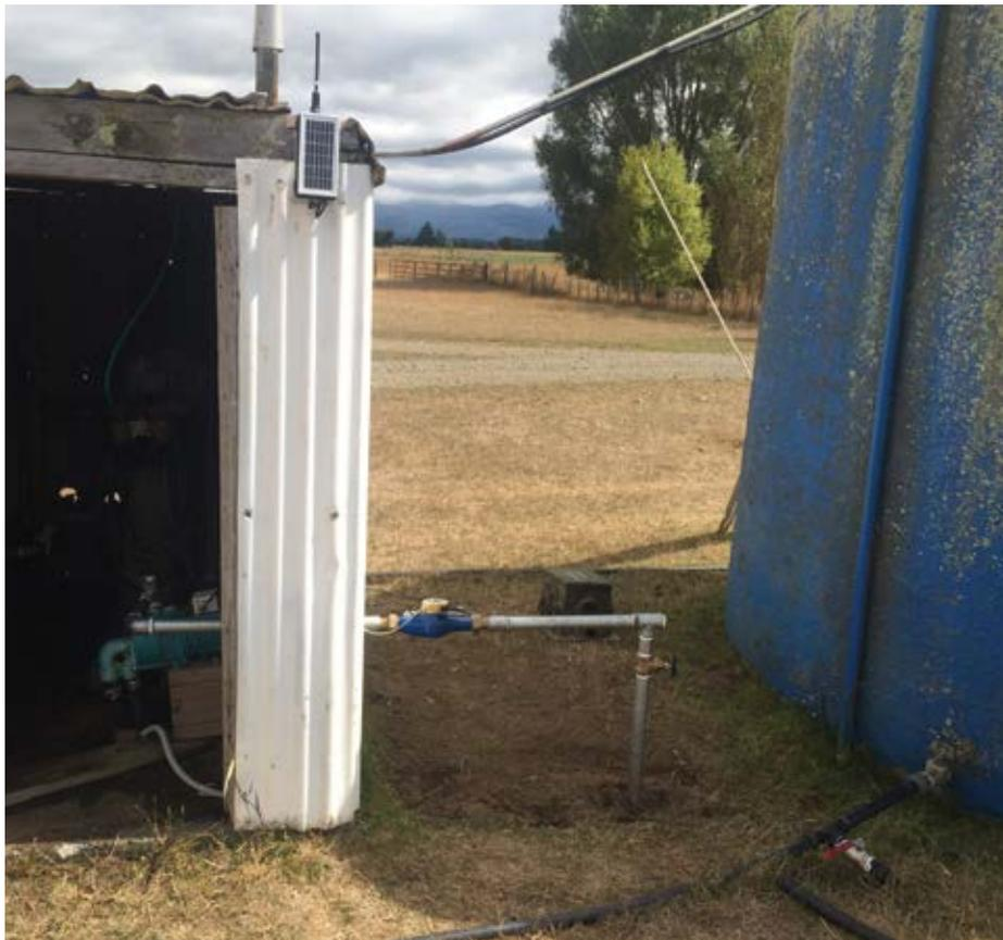
HBRC has an alarm system for all telemetry units. It will email your telemetry provider and the Water Information Services team if we haven't received your data for 48 hours. We set that time limit because most telemetry companies only send in data once a day, so if one transmission is missed, the data can be picked up the next day without loss. After two missed transmissions, HBRC becomes interested. Telemetry companies also have set alarms to track failed sites.
