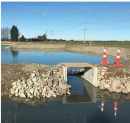
The sediment pond used for holding the water before it flows into the larger recharge pit. Water for the project comes from the Rangitata River via the Rangitata Diversion Race and Valetta Irrigation Scheme.
